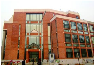
Medical Science Building New Wing, 2013, 193,750 ft 2 /18,000 m 2
